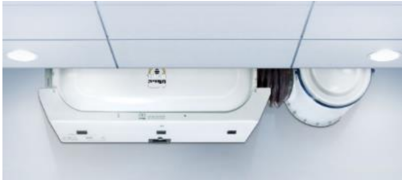
Hidden NBC-Filtration and Ventilation for protection of 30-100 Persons
